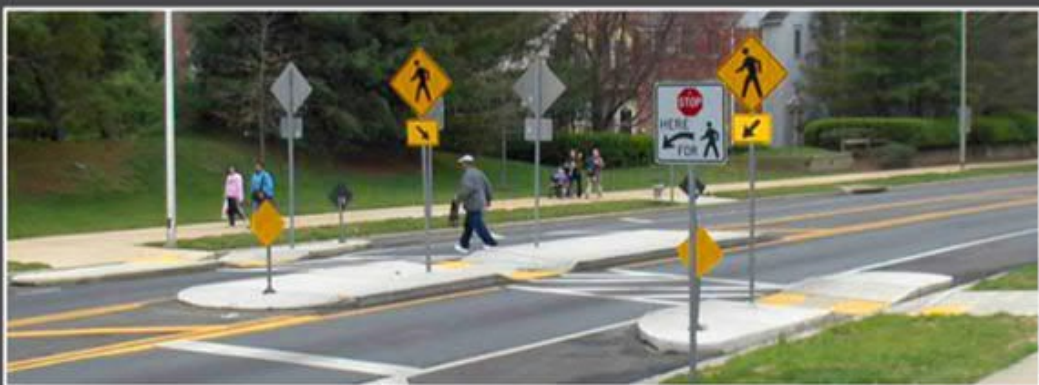
MID-BLOCK CROSSING WITH CENTER PEDESTRIAN REFUGE
